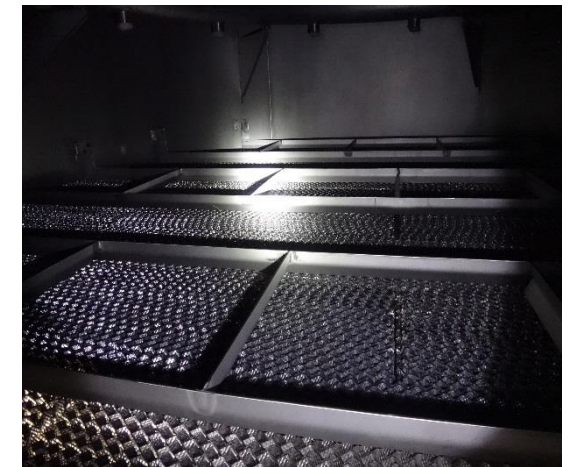
Washwater nozzles and filter inside SOx Scrubber
